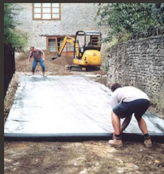
Under aggregate driveway
