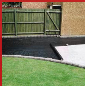
Under Domestic Patio Construction
