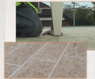
Cover joints with 25mm masking tape...
